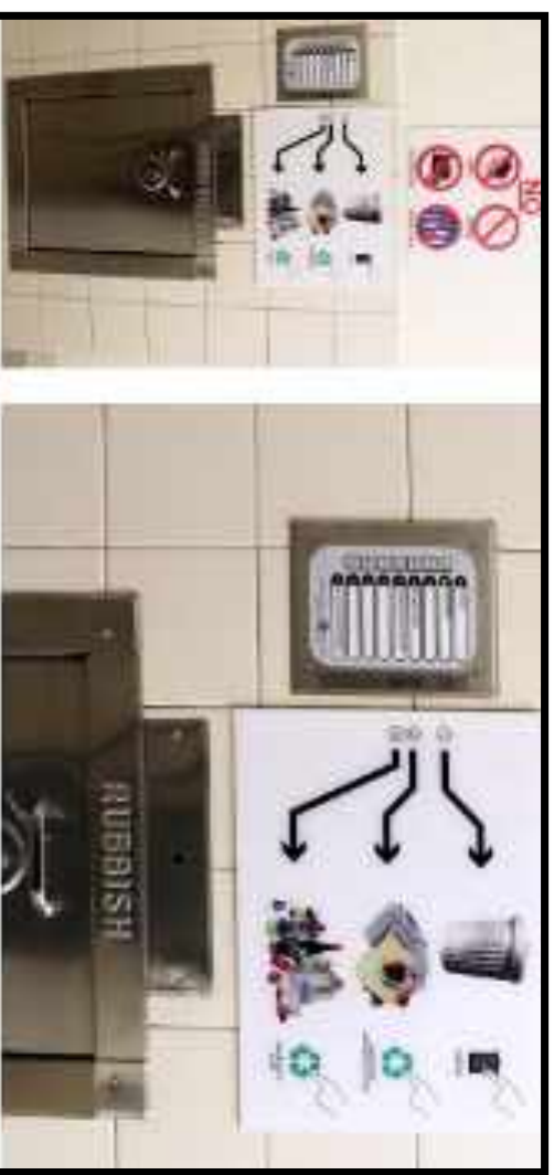
Control panel for residents to select waste streams for binliner and binliner. Chute to 22-Sorter with compactor and binliner.
